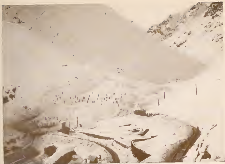
Sewell (El Teniente Mine) in the Snows of June.
